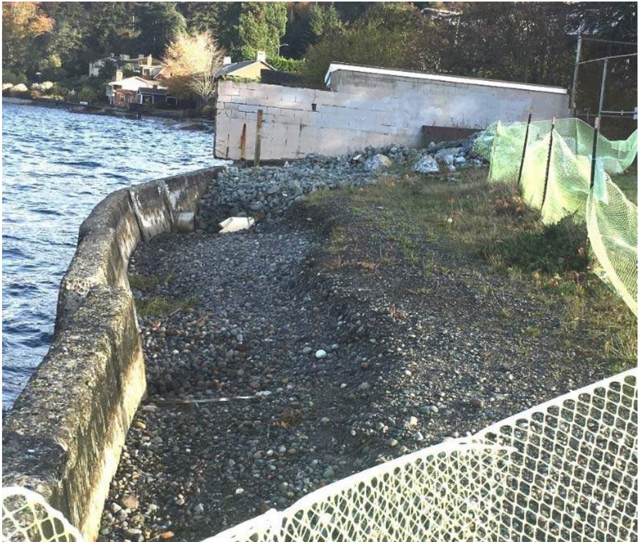
Figure 1. Failed Seawall (Photo taken on 10/18/2016).
