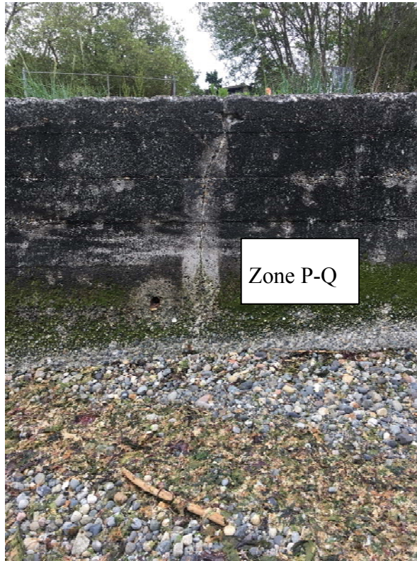
Photo 27. Zone P-Q. Source: Reid Middleton Site Visit 5/31/2017
