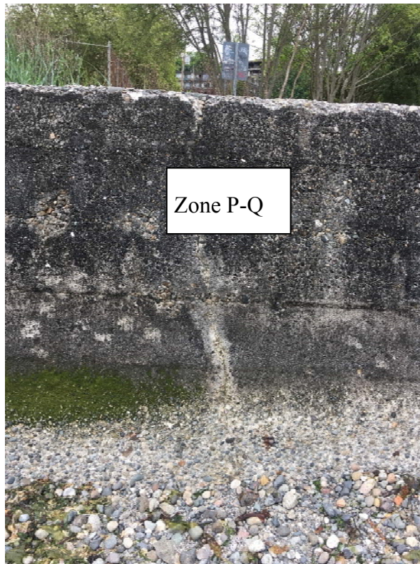
Photo 28. Zone P-Q. Source: Reid Middleton Site Visit 10/18/2016
